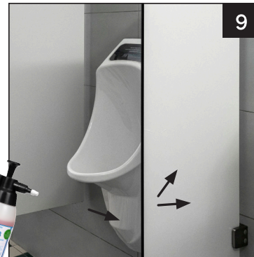
Wipe the lower part of the urinal and its surroundings.
